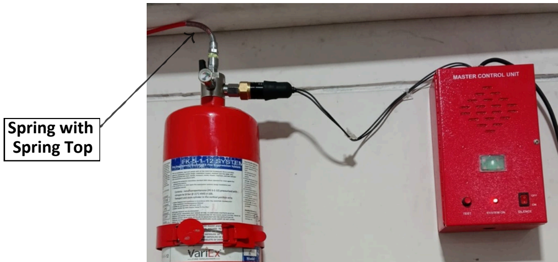
Spring with Spring Top Used in Cylinder Valve Actuation Mechanism.
